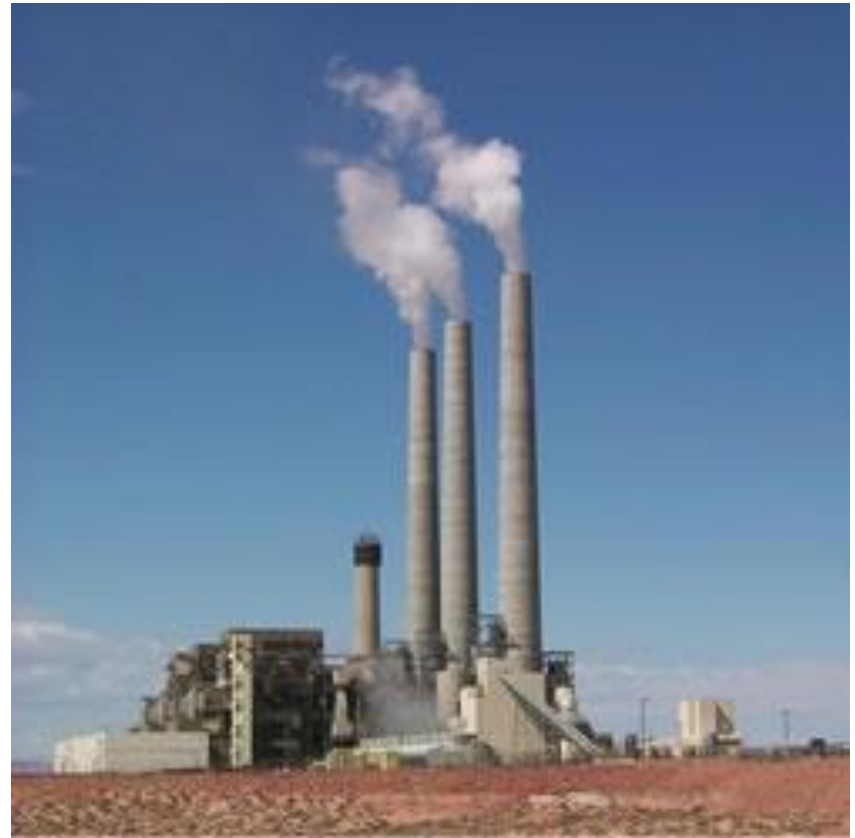
Navajo Power Plant
